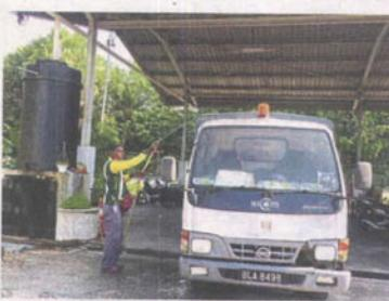
A Solid Waste Management Department worker washing a lorry with rainwater collected from a rain harvester.
